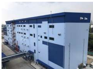
Completion of a nylon yarn production plant for TIAF's airbags on the grounds of IPI
