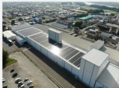
1,608 solar panels (power output approximately 500kW) installed on the rooftop of Inuyama Plant
