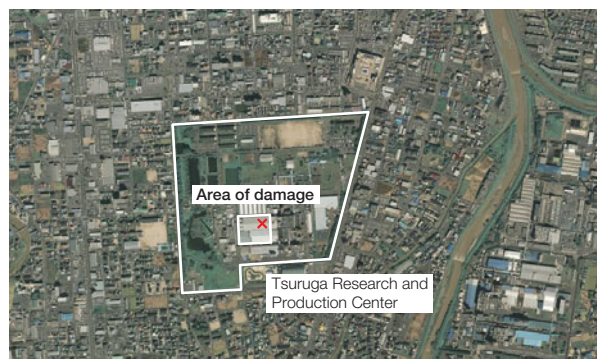
Aerial view of Tsuruga Research and Production Center (Source: Geospatial Information Authority of Japan; compiled by TOYOBO)
