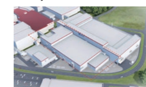
Integrated production plant for CTA dialyzers
