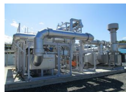
VOC emission treatment equipment
