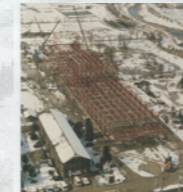
1982 Construction of Nippon Magphane's the Tsuruga Plant
