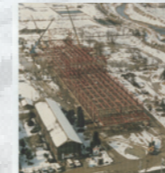
1982 Construction of Nippon Magphane's the Tsuruga Plant
