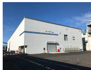
Coating equipment for mold releasing film for MLCC Tsuruga Films Plant Coater Building
