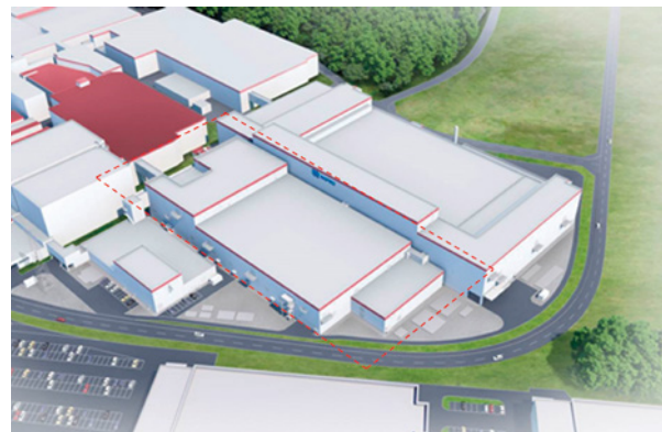
Integrated production plant for dialyzers
