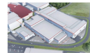
Integrated production plant for CTA dialyzers
