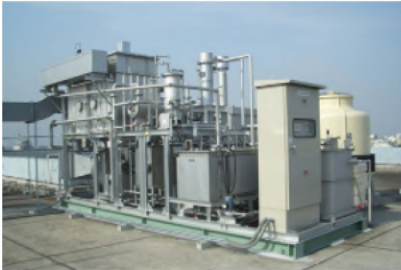
K-FILTER® equipment for VOC emissions treatment
