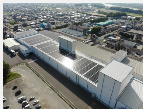
1,608 solar panels (power output approximately 500kW) installed on the rooftop of Inuyama Plant
