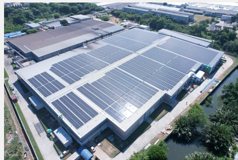
Solar panels installed on the roof of TSSW with a power generation capacity of approximately 2,300 kW.
