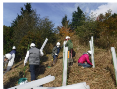
Putting covers preventing feeding damage by deer on saplings
