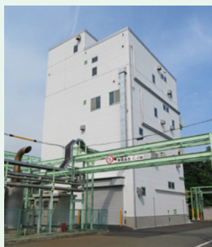
New HARDLEN® manufacturing facility at the Takasago Plant
